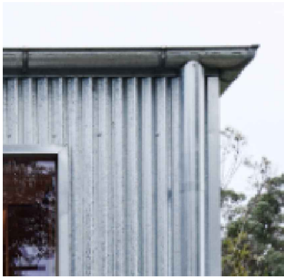
CD-1 VERTICAL ZINCALUME CORRUGATED CLADDING
